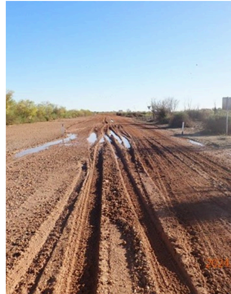
81A Eyre Developmental Road – 2024 flood damage.
