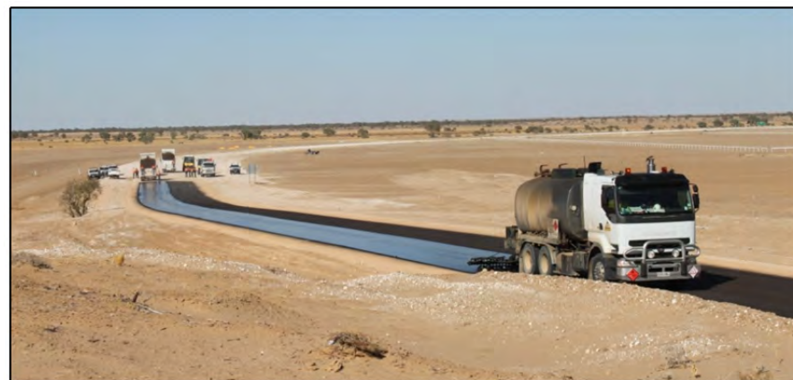
Bitumen sealing on the Birdsville to Windorah Road
