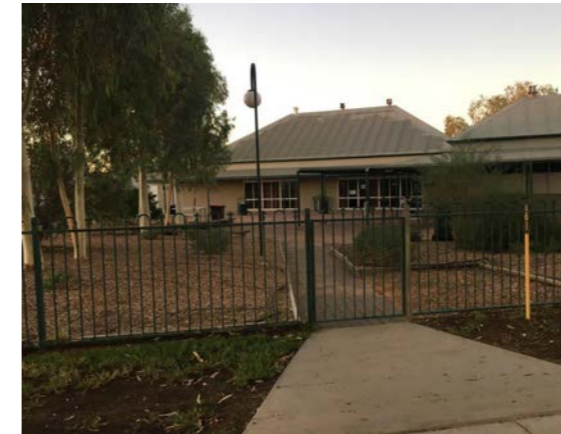
Upgrade to entry required to improve amenity, visual cues and function.
