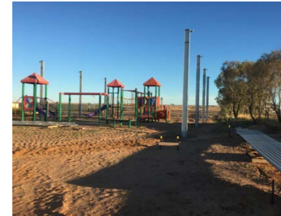
Playground & shelter under constructio.
