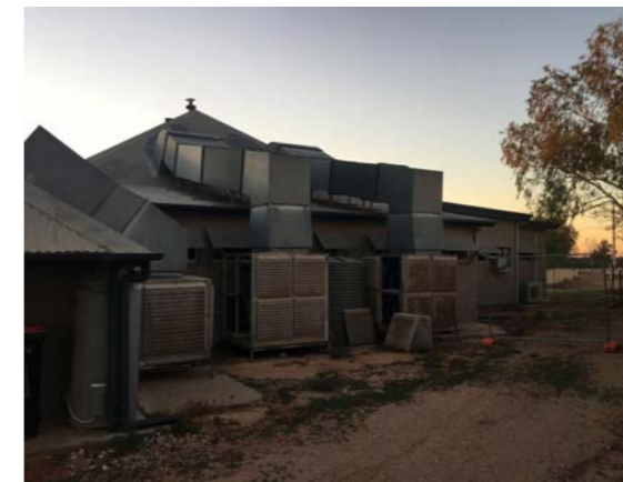
Building Services Area.
