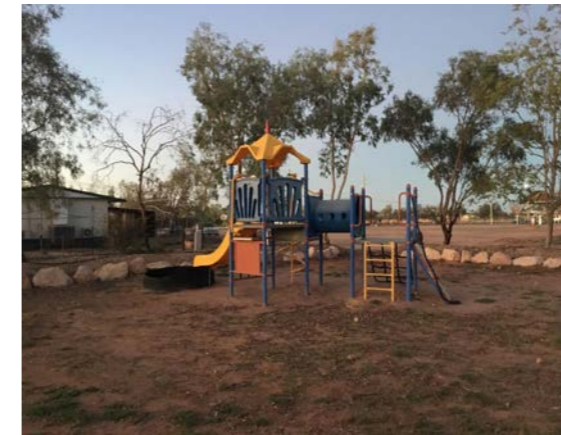
Playground needs soft fall and revised garden layouts to meet safety standards.
