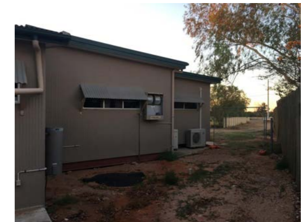
Building Services Area.
