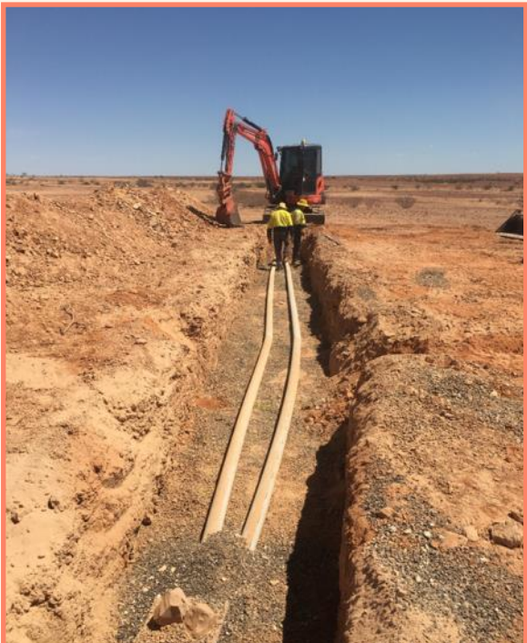
Slotted pipe in transpiration trench
