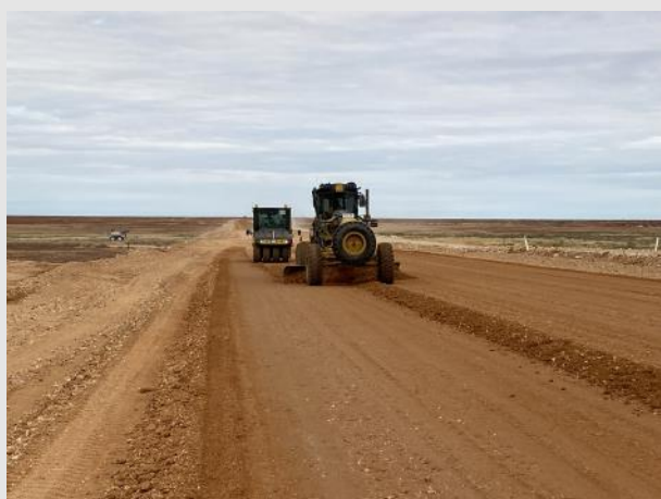
Figure two: Heavy formation grading
