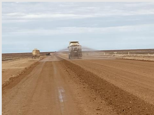
Figure one: Heavy formation grading
