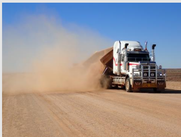
Figure three: Gravel re-sheeting
