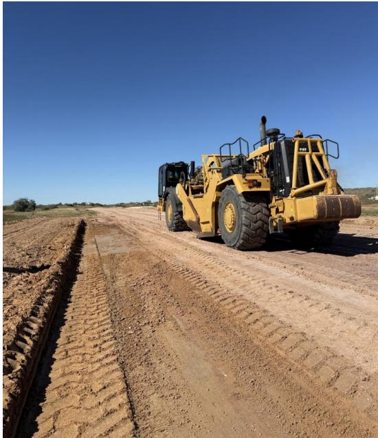
Boxing out soft spots at the Industrial Estate.
