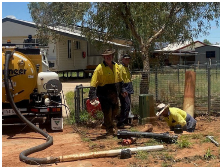
Staff working to repair the blown fire hydrant in Bedourie
