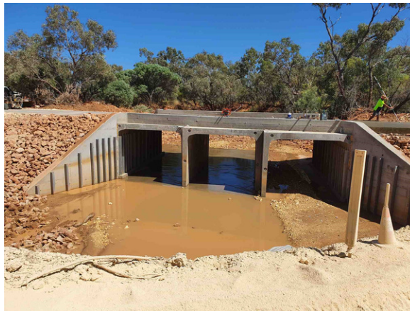
Completed culvert
