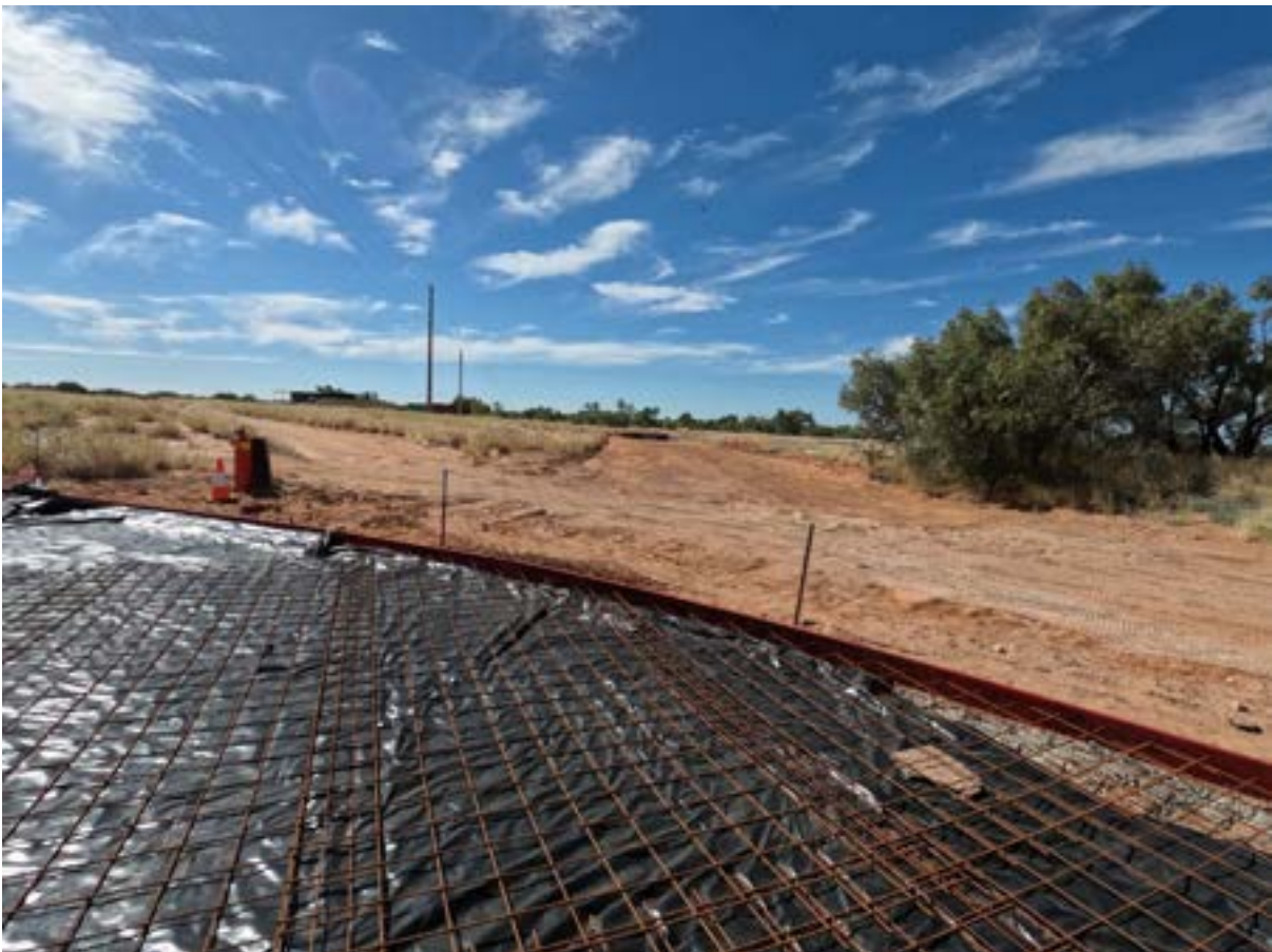
Figure 2 Concrete floodway and culvert inlet which will be rock lined
