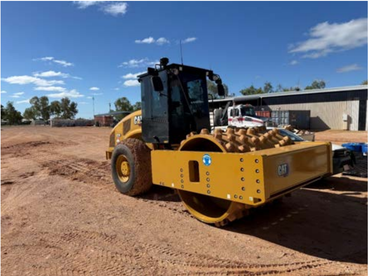
New CS19 cat roller ready for work
